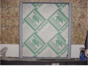
Replace two anchors on the sill and two anchors on the head with a 12mm x 40mm flat hex socket screw to hold the window in place while removing the side tubes.
