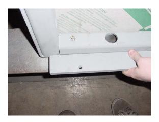
Remove the anchor bolts holding in the head and sill 2" tubes. There are two 6mm flat head machine screws holding the steel tube to the window. If reglazing a teller window the sill will have two flat hex socket screws holding the sill bar in place. These screws (and bolts in the case of a teller window) are used to keep the tubes in place while installing the anchors. Remove these screws also. Remove the head and sill tubes.
