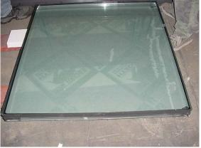
Proceed to the opening and center the glass in front of the setting blocks equally in the opening. Raise the panel up while maintaining on the setting blocks making sure you do not touch the butyl. Touching the butyl can move your glass out of position.
