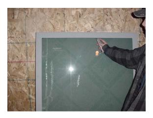
Once the glass has been removed, clean the excess butyl from frame. Re-apply new butyl to the window frame by holding it back 1/8" from edge along all sides except the bottom of the vision opening. The bottom should remain flush when you apply the new butyl. The butyl will spread and overlap the frame or end up flush with the edge of the frame.
